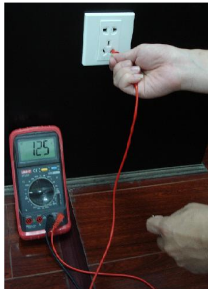
Appendix Figure 7-6 Live cable
