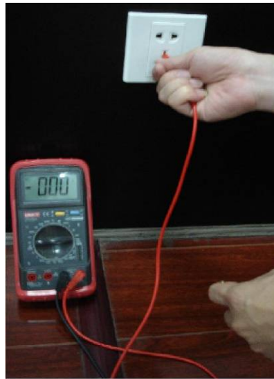
Appendix Figure 7-5 Earth cable
